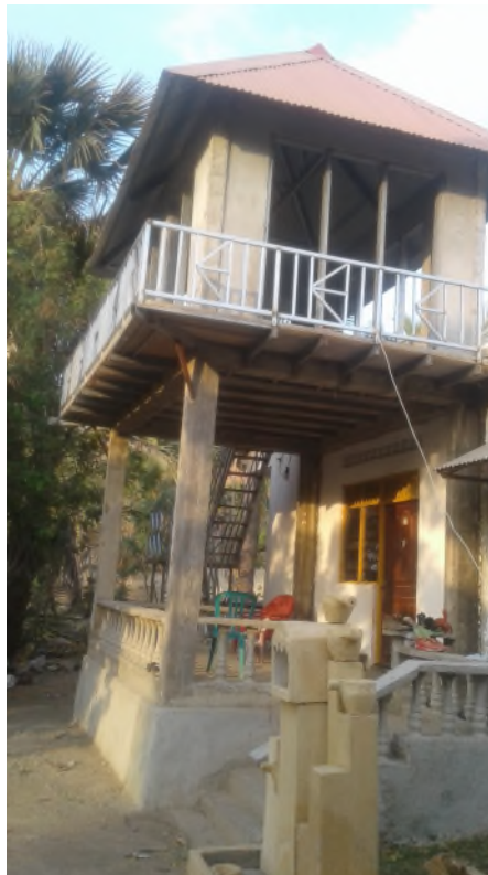
Extensions to the office at Tasitulo
